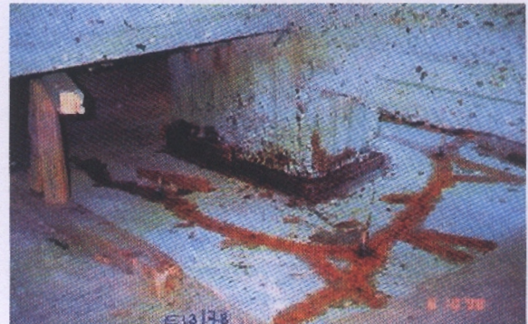
Foundation and column neck injection
