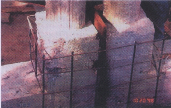
Section enlarged steel bars
