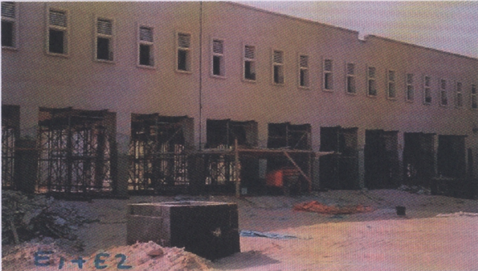
Steel Propping For Beams and Slab
