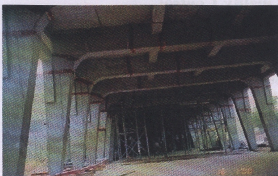
Injection of main frame
