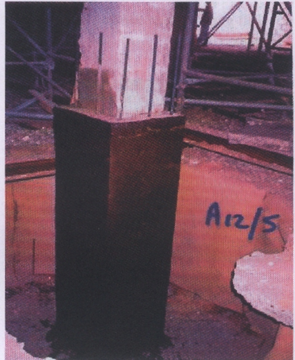
Concrete Jacketing and surface applied protection
