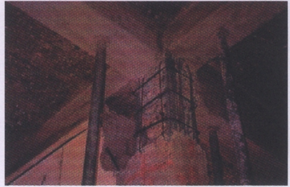
Cut back deteriorated concrete at the soffit of beams
