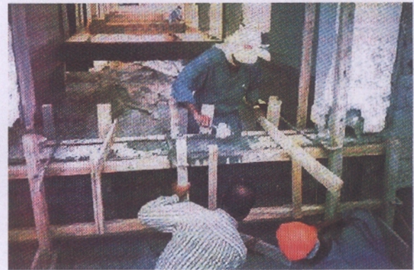
Casting repair material
