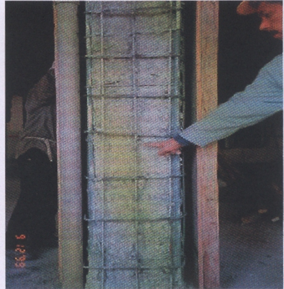
Formwork for sides of columns
