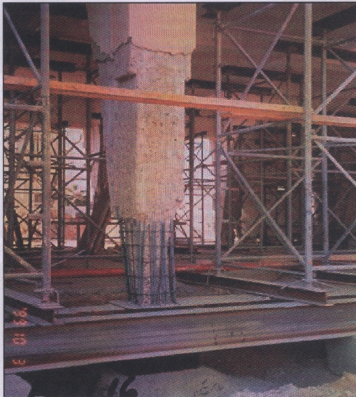
Steel Propping For Column Repair
