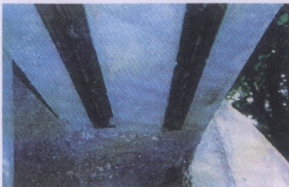
Application of CFRP to brick walls and concrete girders
