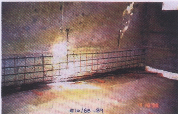
Preparation for ground beam injection
