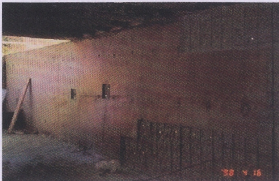
Cutting back to expose the surface area of walls
