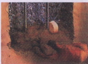
Fixing of zinc anode to concrete surface
