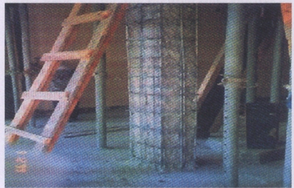
Removal of deteriorated concrete above slab level
