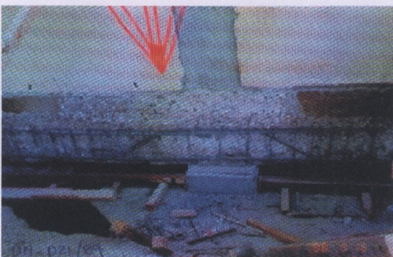
Prepare Tie Beam for section enlargement
