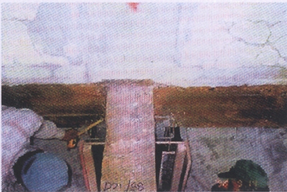
Removal of form work
