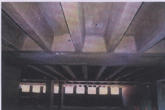
Ribbed Beams after repair
