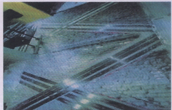
Application of CFRP to brick walls and concrete girders
