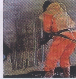
6. Clean Reinforcement
