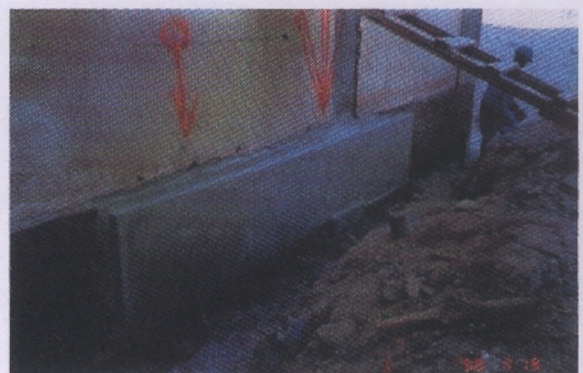
Tie Beam Jacketing after completion
