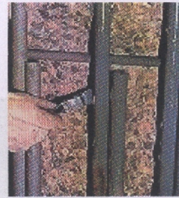
8. Prime Reinforcement
