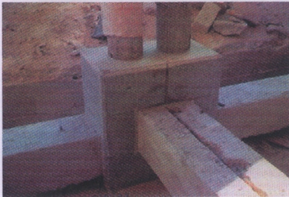
Column neck after repair
