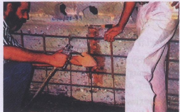
Injection of ground beam
