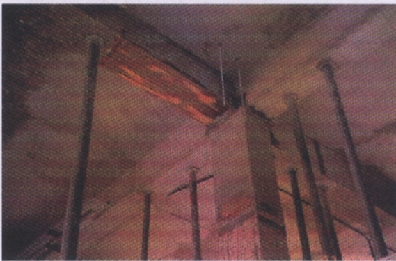
Column after repair
