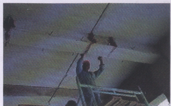
Injection of suspended beams
