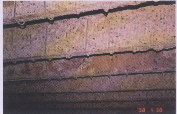
Removal of all deteriorated concrete and sand blast all exposed surfaces
