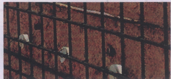
Placing of zinc anodes
