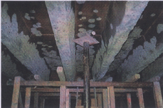
Delamination of concrete cover after fire damage
